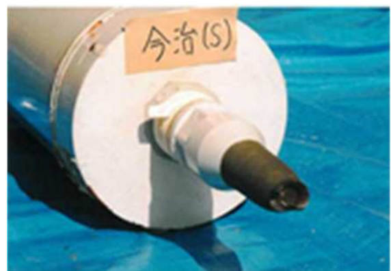
Photo.3 Breakage of the center stay rod caused by the Geiyo earthquake in 2001
