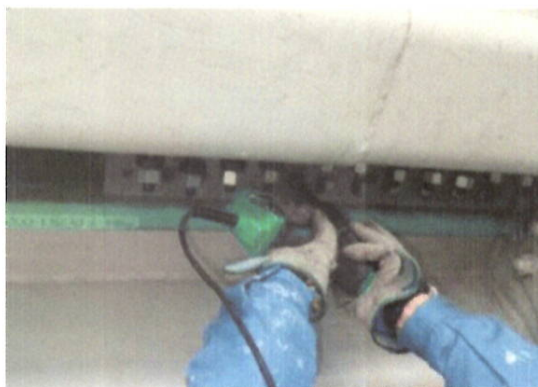
Figure 9. Tightening TRS \phi 16
