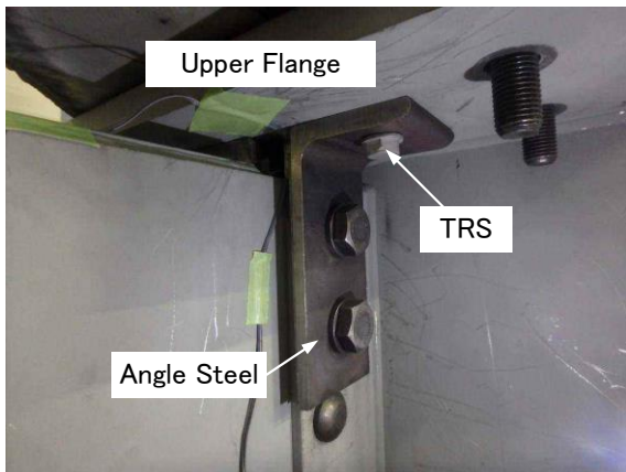
Fig.4 Angle Steel Retrofitting Method Using TRS
